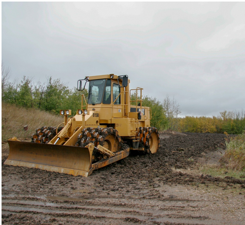
Figure 1. Machinery preparing the BNLO site in September 2006. Photo by Rick Bramm.
